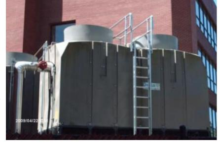
either stainless steel or galvanized metal clad models, which will eventually rust and corrode," Alkarmi says. "The Delta HDPE design does not require any coating or galvanizing or other exterior protection. It simply will never rust or corrode, and will last well over 20 years."
